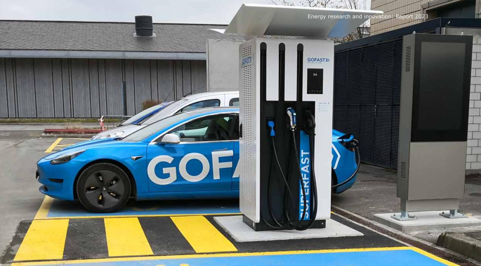
Within 15 minutes, the fast-charging station on the EPFL campus can supply two electric cars with enough electricity to drive 100 kilometres (source: MESH4U).
