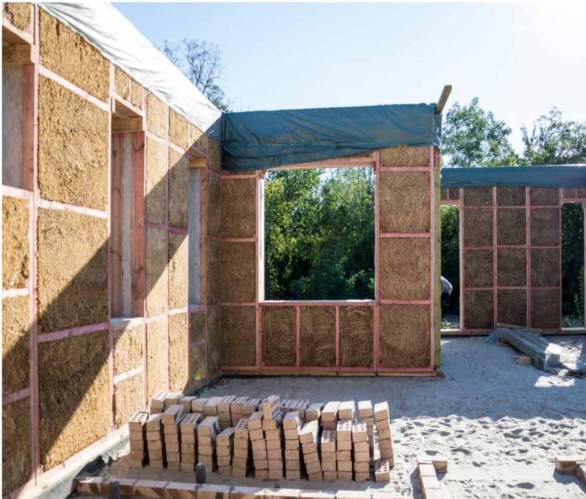
Lightweight construction, such as the wooden frame construction with straw insulation shown here, generally has a lower impact on the climate and environment than solid construction with ceramic or mineral building materials such as bricks or concrete (source: Shutterstock).
