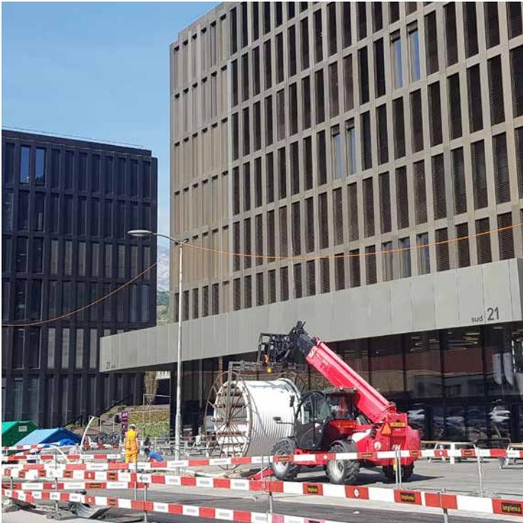
The white pipes were laid underground from the coil and now transport the CO<sub>2</sub>. Thanks to the smaller cross-section compared to water pipes, fewer deep excavation pits had to be dug (source: HES-SO Valais-Wallis).
