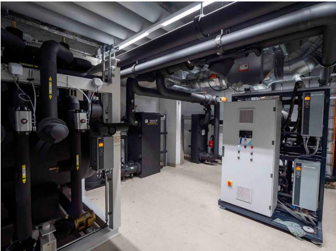
In the energy centre of the energy network, the groundwater cools or heats the CO<sub>2</sub> via a heat exchanger (source: HES-SO Valais-Wallis).
