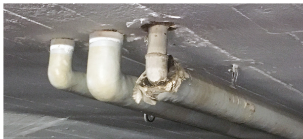
Repair defective heat insulation.
