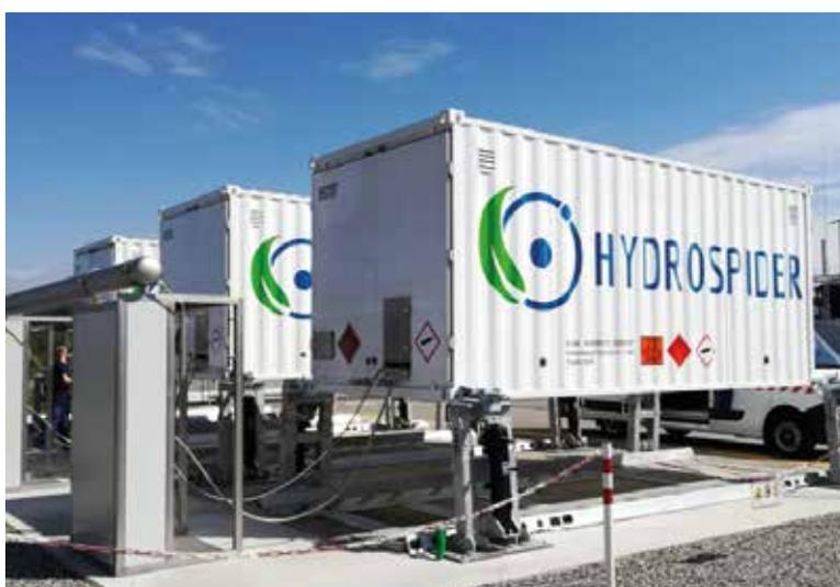
A 2MW electrolyser plant at the run-of-river power plant "Gösgen" will go into operation in 2020 to produce "green hydrogen" for fuel cell trucks. The picture shows tank containers, where the hydrogen produced is temporarily stored and which are used to supply the filling stations in Switzerland with hydrogen (Source: HydrosSpider).
