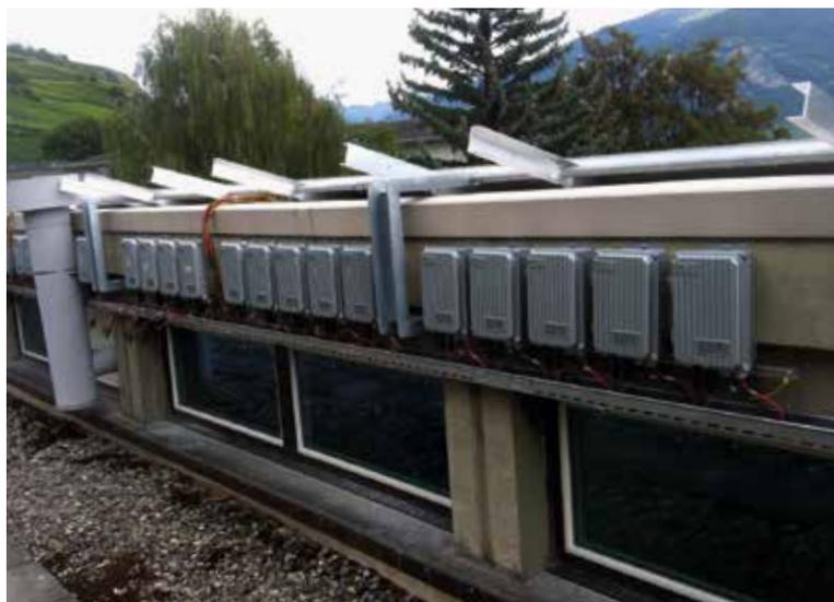
DC/DC converter for individual photovoltaic modules on the roof of the HES-SO Valais Wallis. Each of the 45 modules is connected to the DC bus via its own converter with integrated maximum power point tracker. The efficiency of the individual converters is 97 to 98 % (source: HES-SO Valais Wallis).
