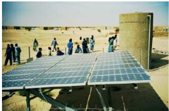
Solare Wasserpumpstation in Mali
